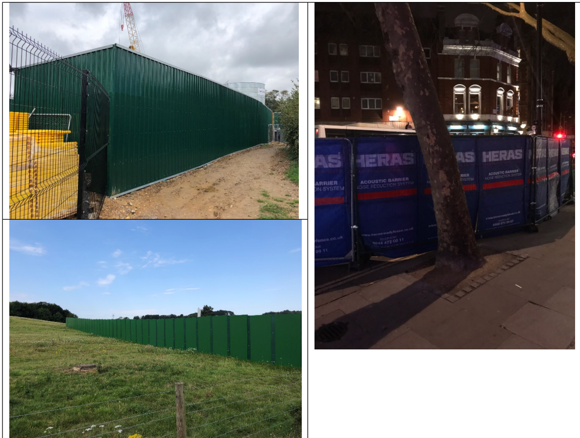
Plate 6.1 – Example noise screening solutions
